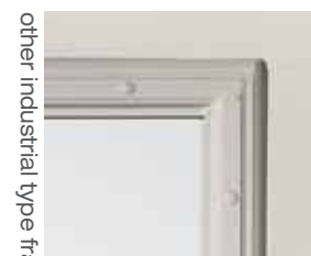
The width of most industrial type frames limits your choice of locksets, and they have industrial looking profiles.
